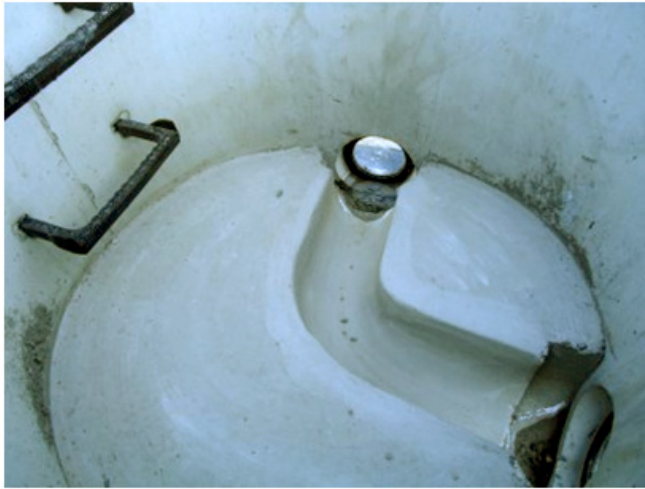
Typical bench layout before installation.
